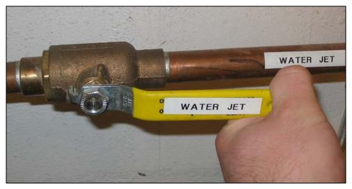
Figure 33 Turning water on/off to water jet cutter
