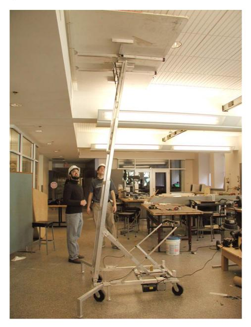
The drive mechanism is the small black motor seen attached to the base. The extensible lift was tilted slightly backward, so that as the drywall was lifted, it brought
