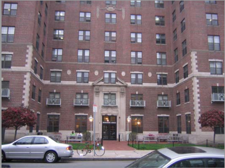
Figure 1: Large Hotel Apartment Structure. Today it is a BU dorm. The Sheraton can be seen engraved over the door, a trace of the past.
