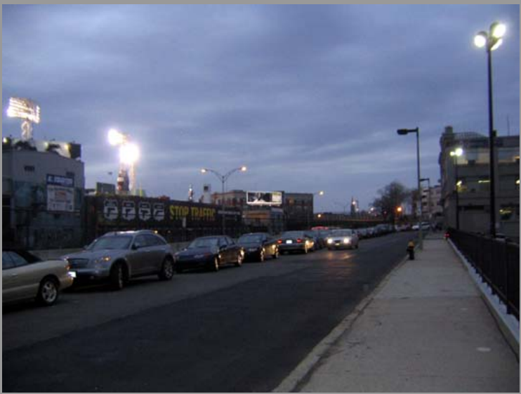
Figure 16: The interstate occupying the site where the old post office and other buildings once were.
