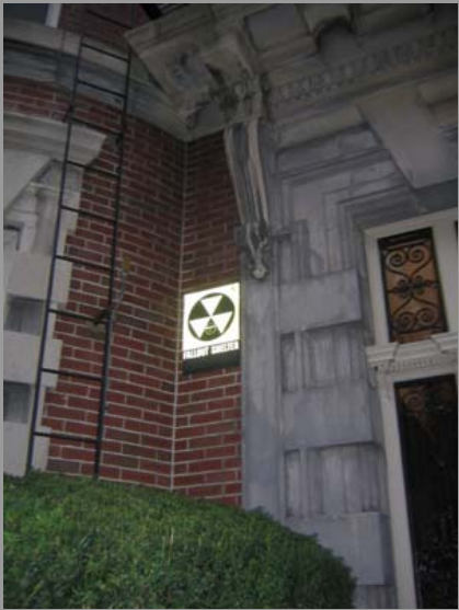
Figure 17: Fallout Shelter sign
