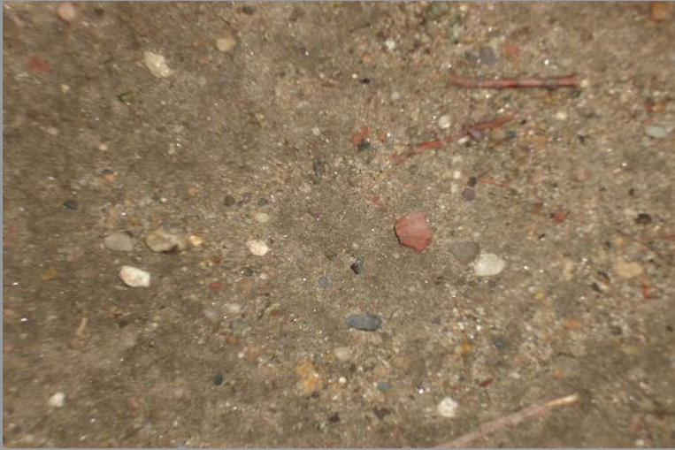
Figure 21: Photo (12) Compacted Soil
