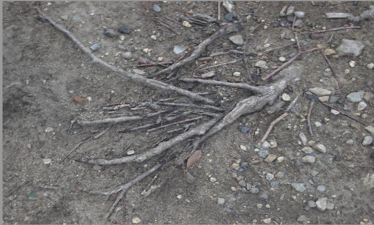
Figure 18: Photo (9) Exposed Roots
