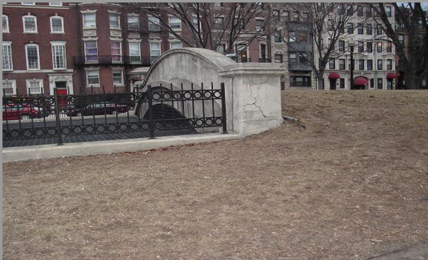
Figure 20: Photo (11) Subway Vent
