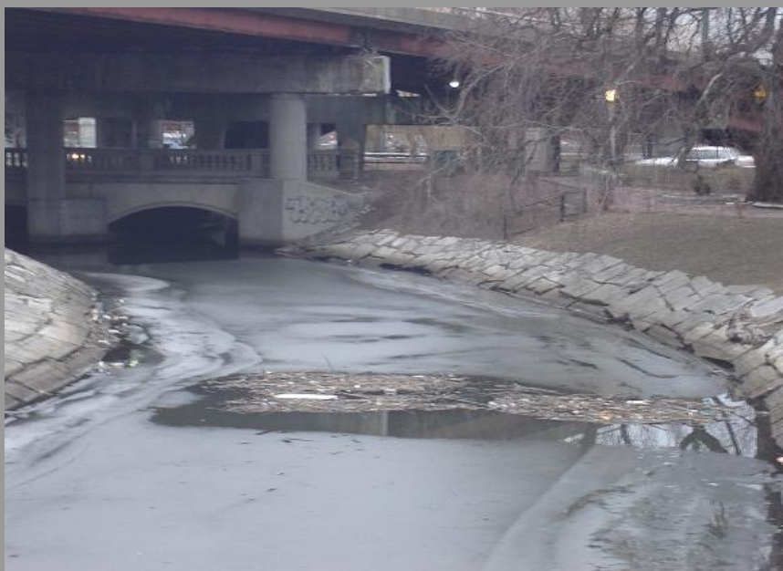
Figure 5: Photo (1) of stone-lined river in Kenmore
