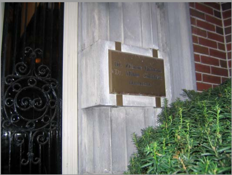
Figure 11: Plaque detailing dentists in the building.
