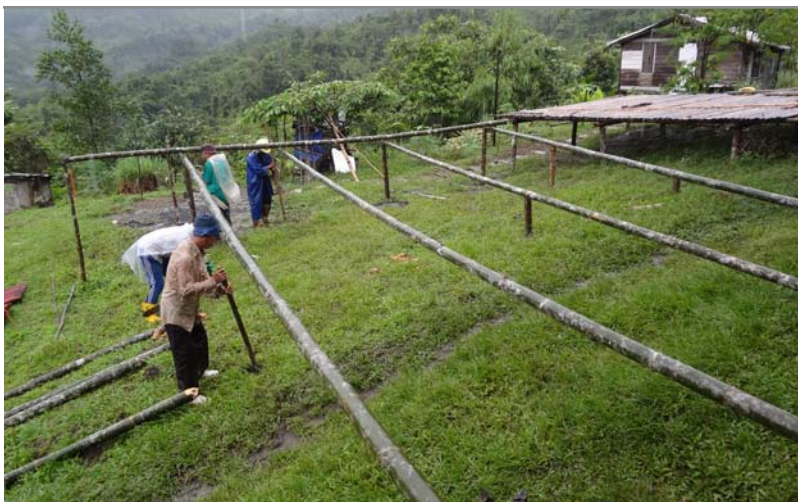
Figure 21. Kampung Rejai villagers building a deck out of bamboo for an upcoming festival. Photo by Jennifer Ly, 2015.
